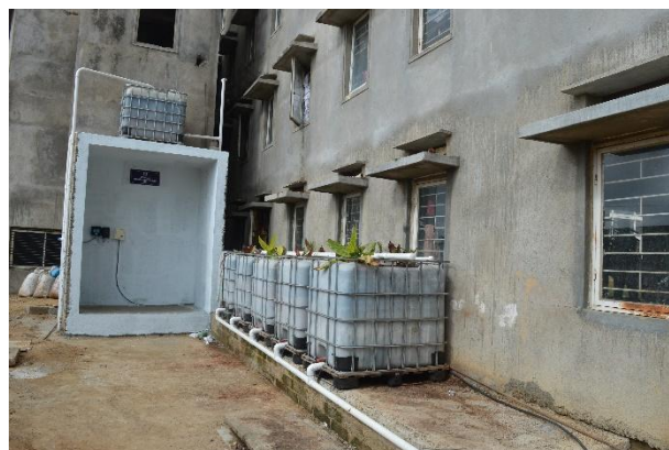
Installation of STP in AMCEC campus
